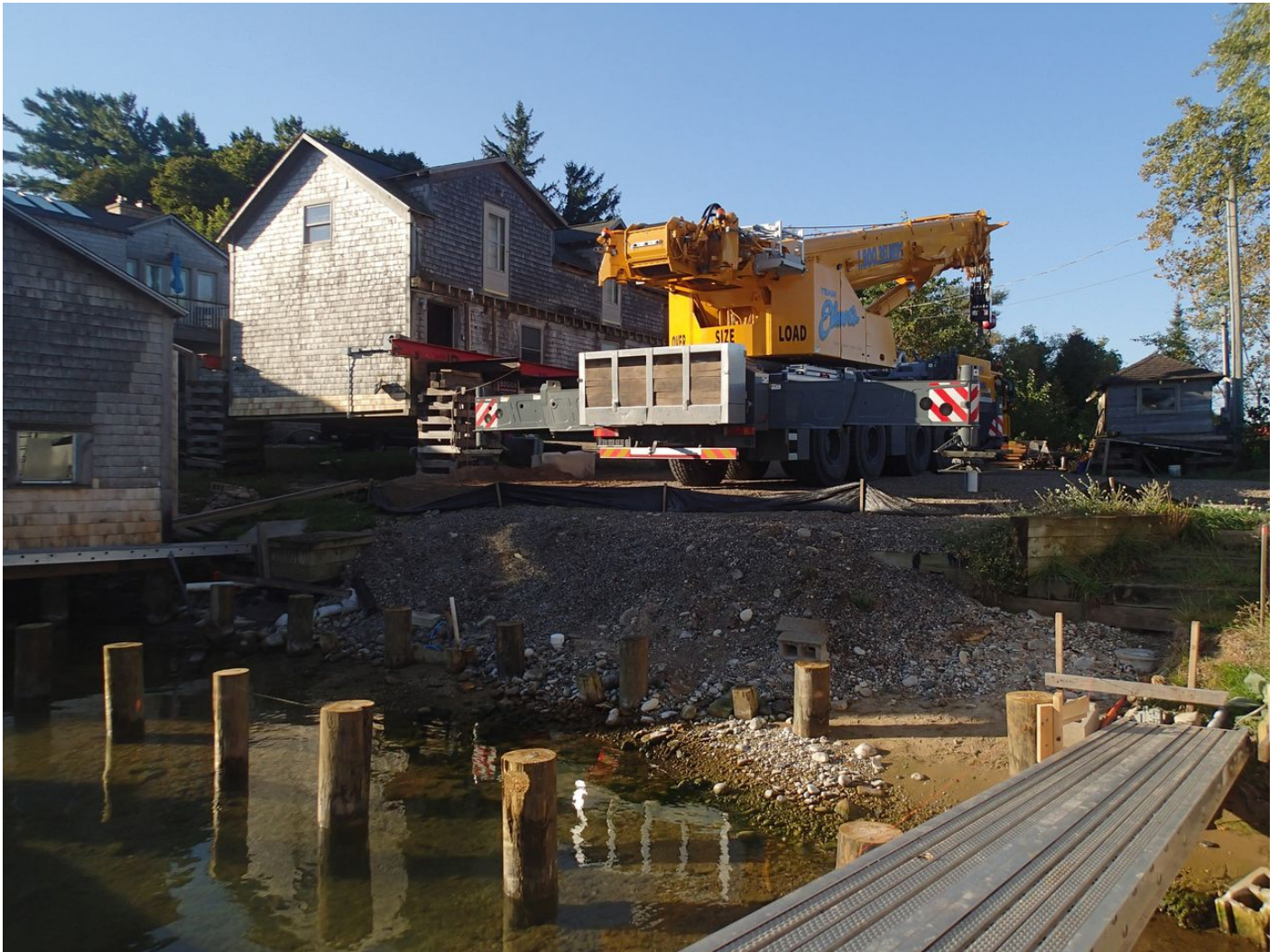
Fishtown's Otherside Shanty was lifted off its old foundation last year and recently returned to a higher, more solid perch. Photo provided by Amanda Holmes.
