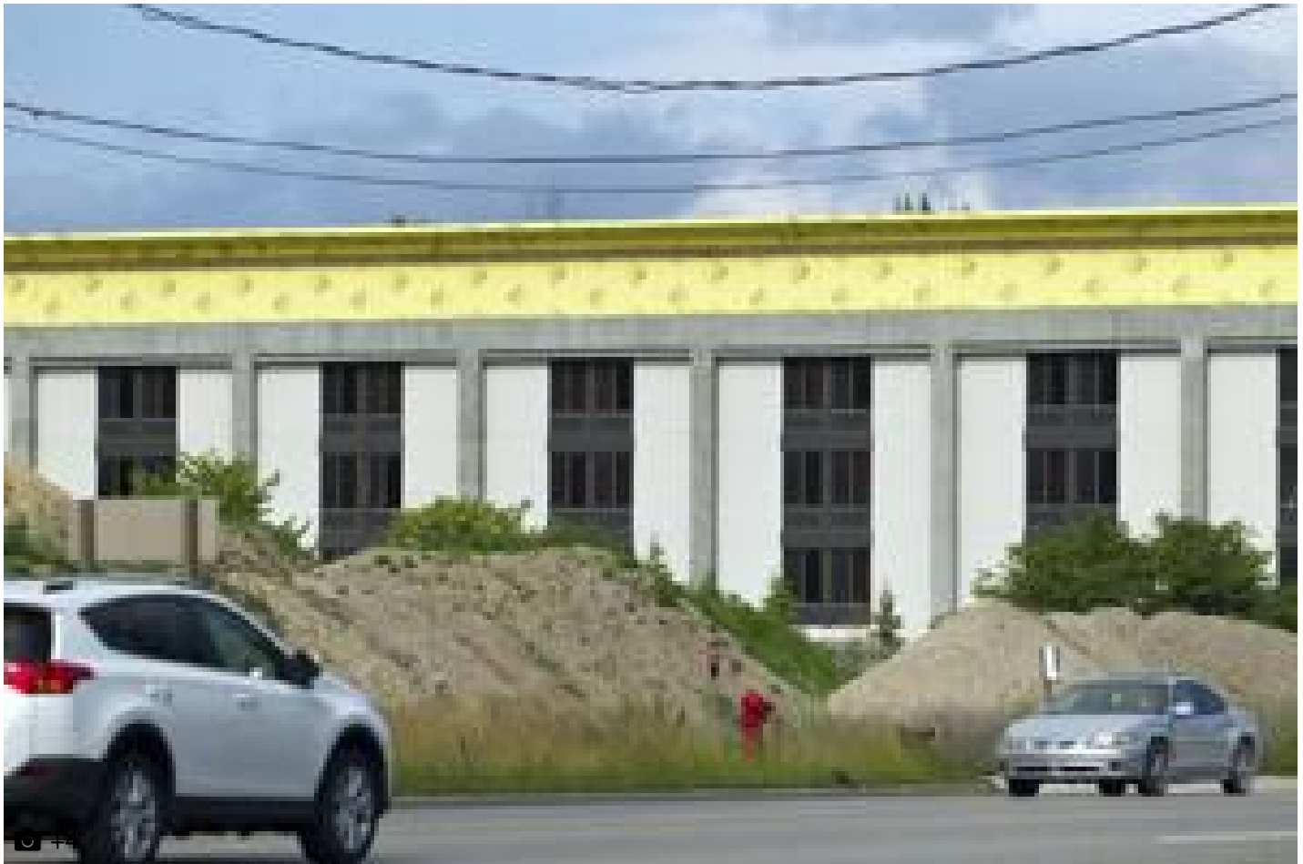
East Bay building boom
