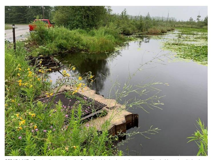
CEDAR LAKE – Construction to replace the Cedar Lake lake level control structure will begin this week and take place over the next several weeks. The decaying structure, originally installed in the 1950s, is in dire need of repair, according to officials.
