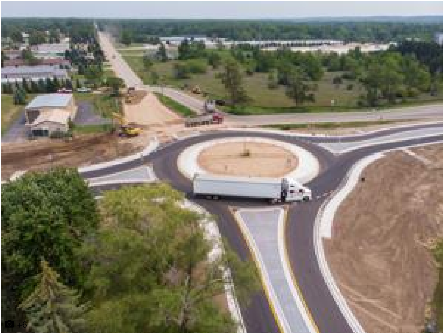
Missing the curve: Tractor-trailer gets hung up in new M-37 roundabout
