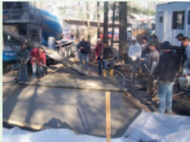
highly permeable, interconnected voids that drains quickly. Pervious concrete allows 3 to 8 gallons of water per minute to pass through each square foot of the material.
