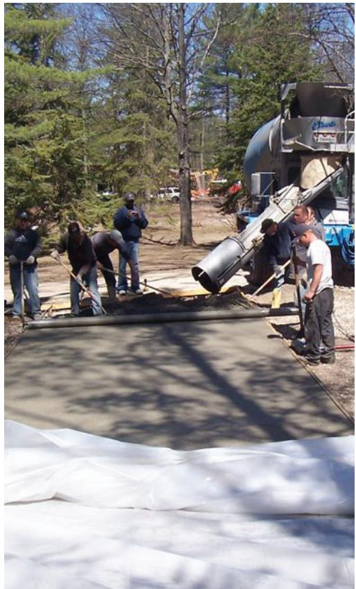
Pervious concrete lets the "river run through it," so to speak, so that rainwater returns to and replenishes groundwater, instead of creating puddles and stormwater runoff, an environmental liability.
