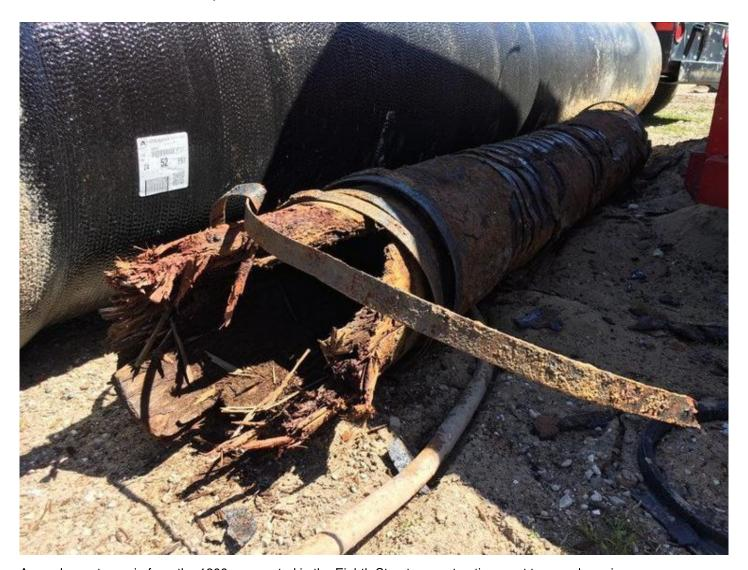
A wooden water main from the 1800s excavated in the Eighth Street reconstruction, next to a modern pipe. Special to the Record-Eagle
