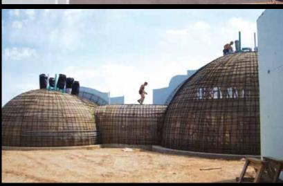
PROJECT: Earth Shelter CHALLENGE: Largest Michigan underground self-sustaining home environment SOLUTION: Shotcrete Concrete Mix with 3/8" peastone for exterior wall
