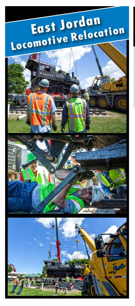
PROJECT: East Jordan Locomotive Relocation CHALLENGE: Lifting the train without damage SOLUTION: Using a rigging loc and attention to detail
