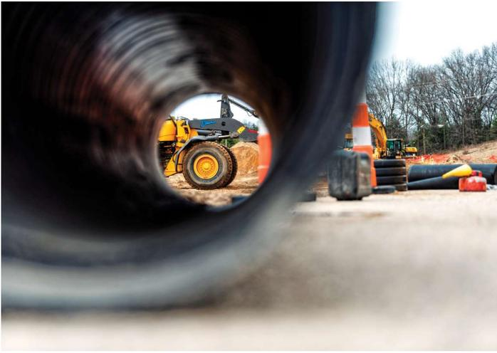
In addition to the 25 feet pipe depth challenge Team Elmer's encountered extra utilities in the excavation scope of work – uncovering three more utilities that were abandoned.
