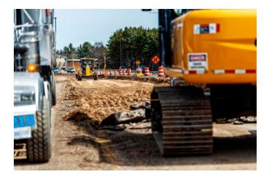
road ranging from six inches to six feet deep underneath the existing asphalt road that had been built over top the concrete. The old road was 20 feet wide and close to the entire length of the project. It was also in the center of the road, which made it difficult for Team Elmer's to allow enough room to maintain traffic on one side while working on the other. Using unique traffic control patterns also helped make the concrete road removal safe and successful.
