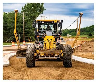
Team Elmer's was able to provide an alternate time line proposal; building both roundabouts simultaneously and condensing the construction schedule to save time. This meant constructing the road in half width increments while maintaining northbound traffic and local access.
